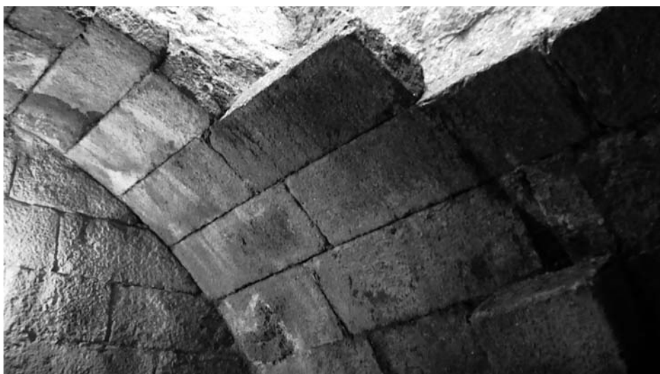
Vista interior aljibe
